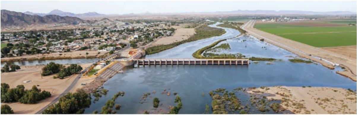
2007 downstream aerial view of Morelos Dam showing normal conditions.
